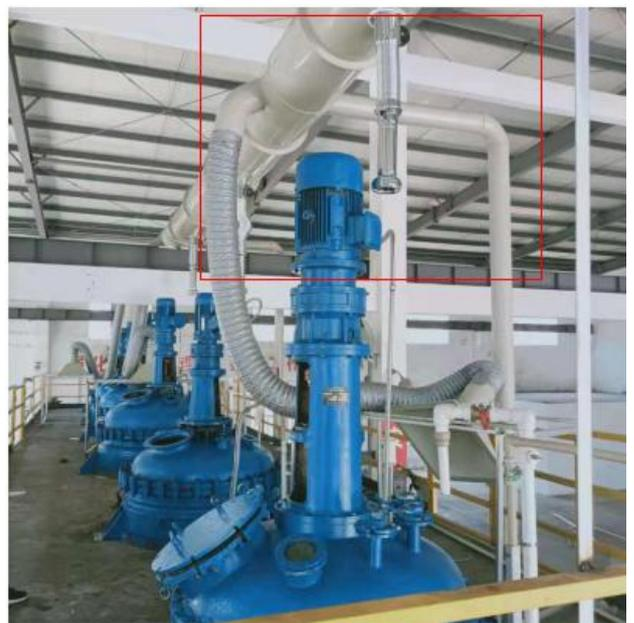
生产废气收集设集气罩
